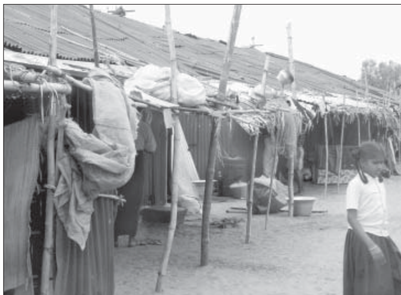
Line housing built of 'tar sheets' at the temporary settlement in Serudhur, Nagapattinam, Tamil Nadu
