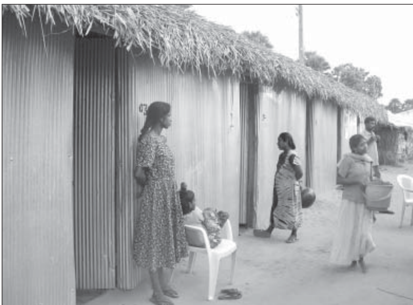
Line housing built of tin and thatch in Kannagigramam (Ampara), Sri Lanka
