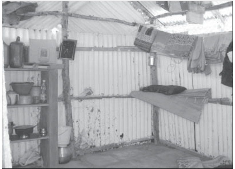
Interior of a temporary housing structure in Tamil Nadu. Most shelters were used to store belongings as the inappropriate material, small size, and intense heat makes them uninhabitable.
