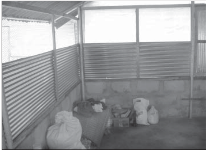
Interior of a TRO shelter at Thiraimadu, Batticalao. The wire gauze fails to provide privacy, while the tar sheet roof and tin walls trap heat.
