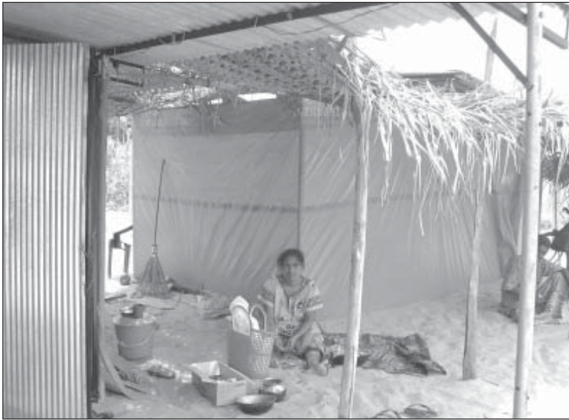
Temporary housing constructed of tin and plastic sheets – Periyaniavalai (Ampara), Sri Lanka. Flooring has not been provided and the shelters are built on the sand. The lack of provisions for cooking forces women to cook outside the shelters.
