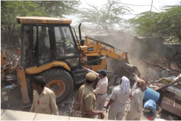
Bulldozers Demolishing Jhuggis, Baljeet Nagar, 24th March 2011
