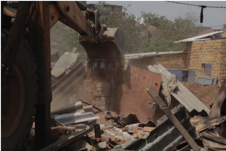
Bulldozers Demolishing Jhuggis, 23rd March 2011
