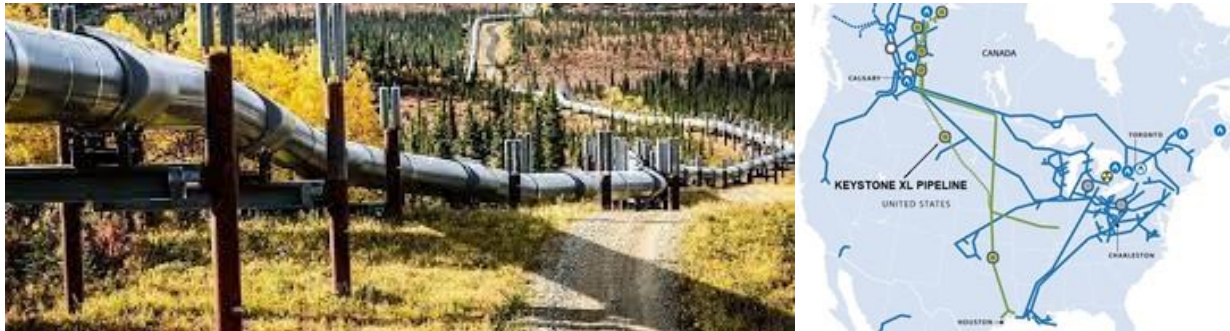
Figure 5: (L) The controversial Keystone XL oil pipeline crossing North Dakota. Source: oilprice.com; (R): Map of Keystone XL Pipeline, a project to move heavy crude oil from the tar sands region of Canada to Nebraska, where it will then move on to refineries in Illinois and along the Gulf Coast. Source: TC Energy
