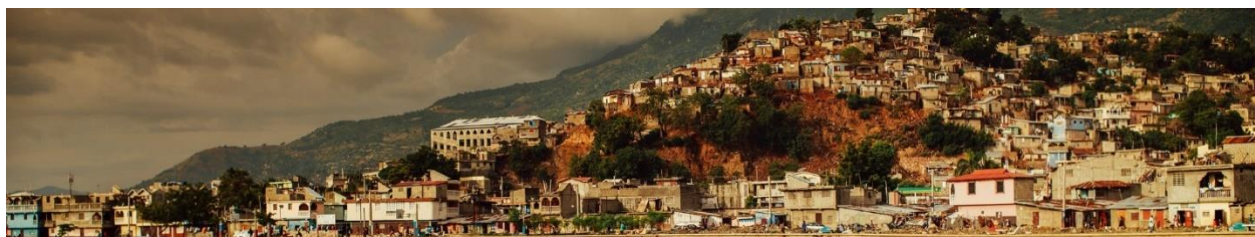
Figure 5: A view of Shada before the demolition. Source: Meds & Food for Kids.
