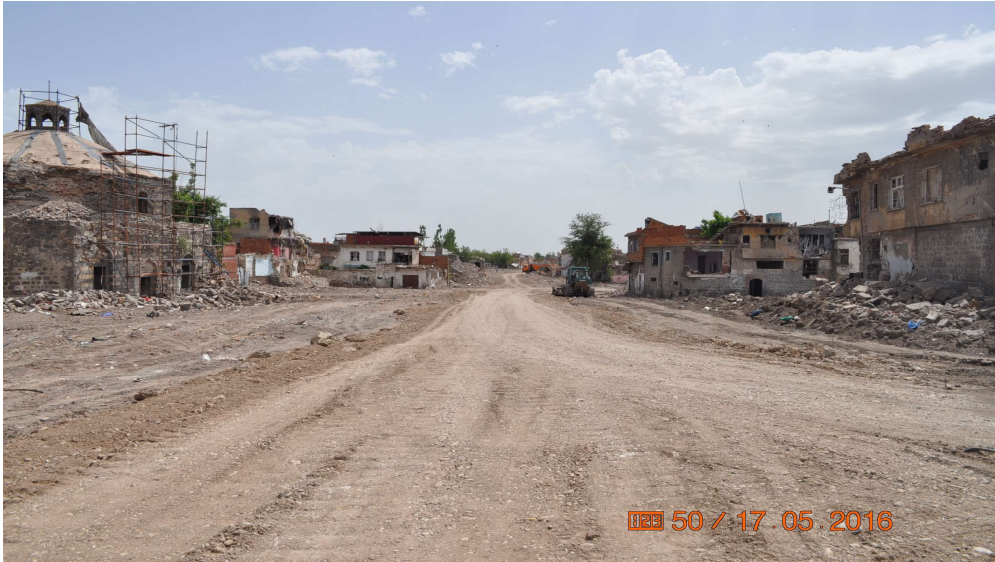
Photo. 9: The Yenikapı street, which kept its original width of 8m before the demolition, has been turned into a 15 m wide street.
