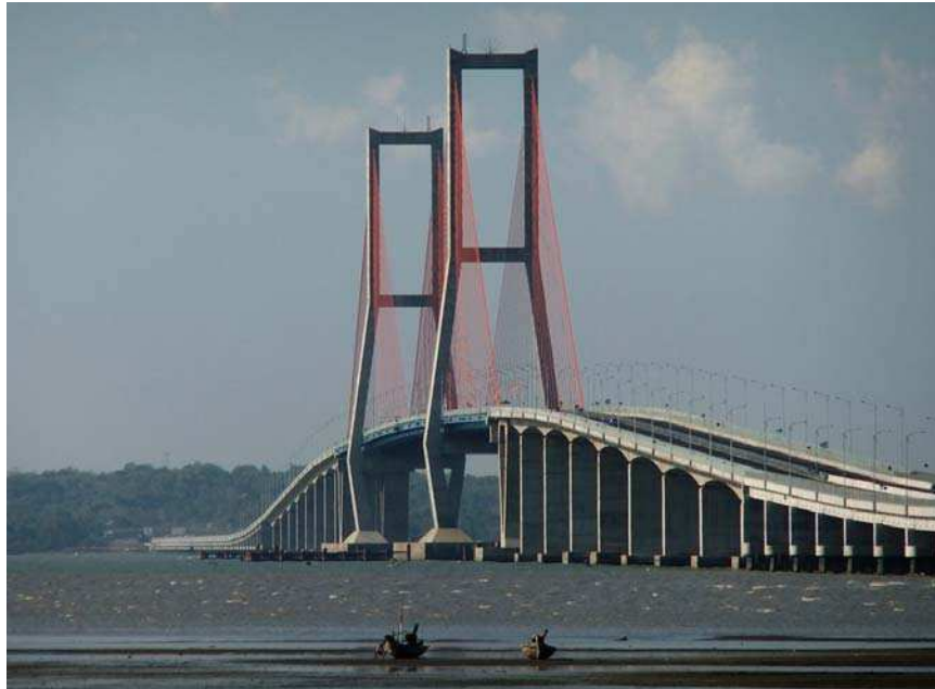
Figure 3-5: Suramadu bridge connecting Java island and Madura island. (Source: Fakultas Matematika, Institut Teknologi Surabaya, 2009)
