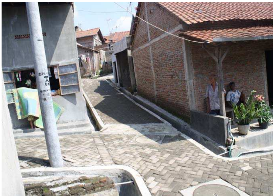
Figure 5-4: Slums upgrading program in Solo. (Source: Surakarta City Government)
