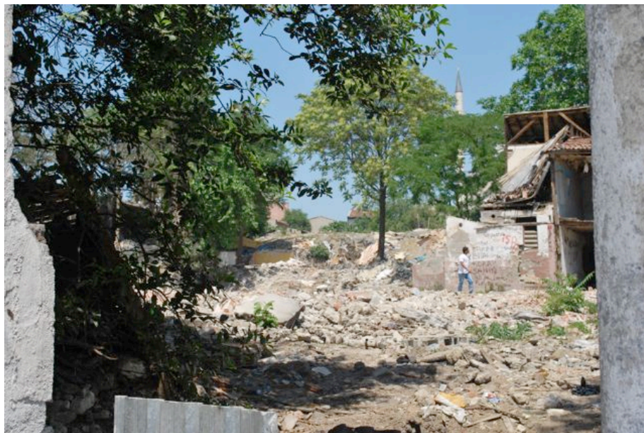
Remains of demolition in Sulukule
