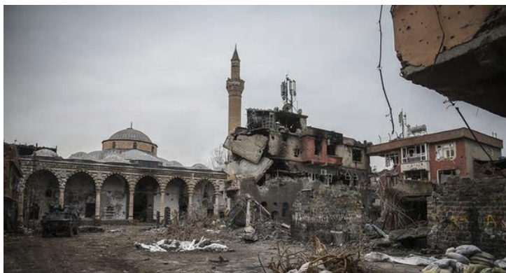
Kurşunlu Mosque in Amed quarter of Diyarbakır, damaged from bombardment by the Turkish military. Source: Fatih Pınar.
