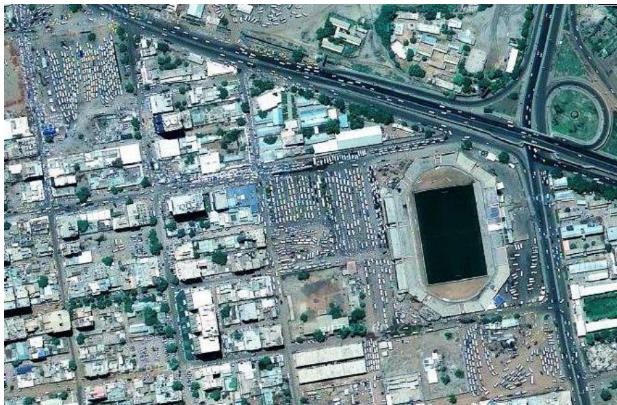
Photo 3: Aerial photo showing new transport terminals near Khartoum Stadium and Jackson Square Source: Worldwide Web
